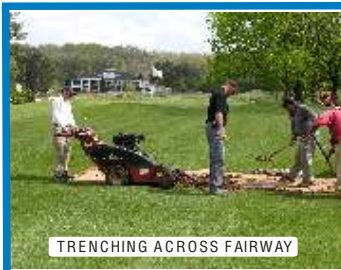
INSTALLING J-Drain / FITTINGS
