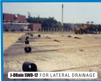
DRAINAGE LATERALS INTO SIDELINE TRENCH
