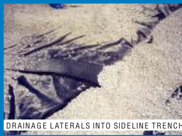
J-Drain SWD-12 FOR LATERAL DRAINAGE
