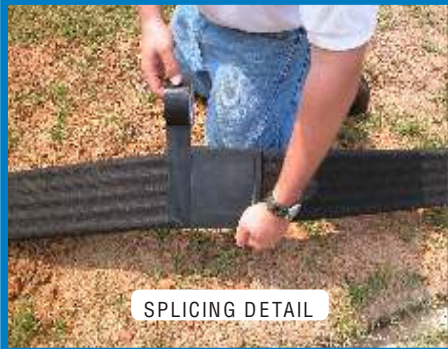
INSTALL AND TAPE FITTINGS
