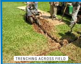
J-Drain SWD-6 IN TRENCH / SAND BACK FILL
