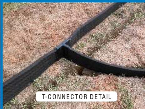
INSTALL AND TAPE FITTINGS
